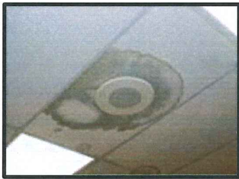
Figure 5: Water Damage - EHS
