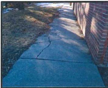
Figure 12: Uneven Sidewalk - FHS
