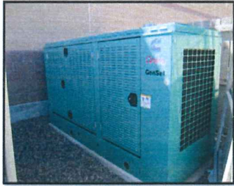
Figure 4: Back-up Generator- EHS
