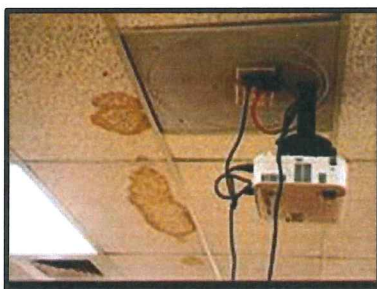
Figure 1: Water Damage - EHS
